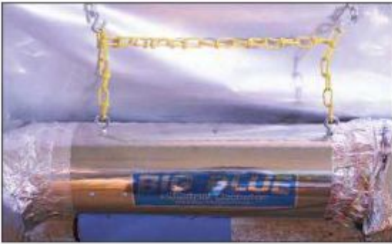
This ozone generator cleans odors as air travels through exhaust tubing.
