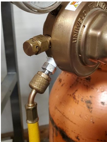
Figure 7-7: Pressure Hose and Nitrogen Tank Regulator Connection
