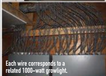
The electrical room was installed by an authorized professional.
