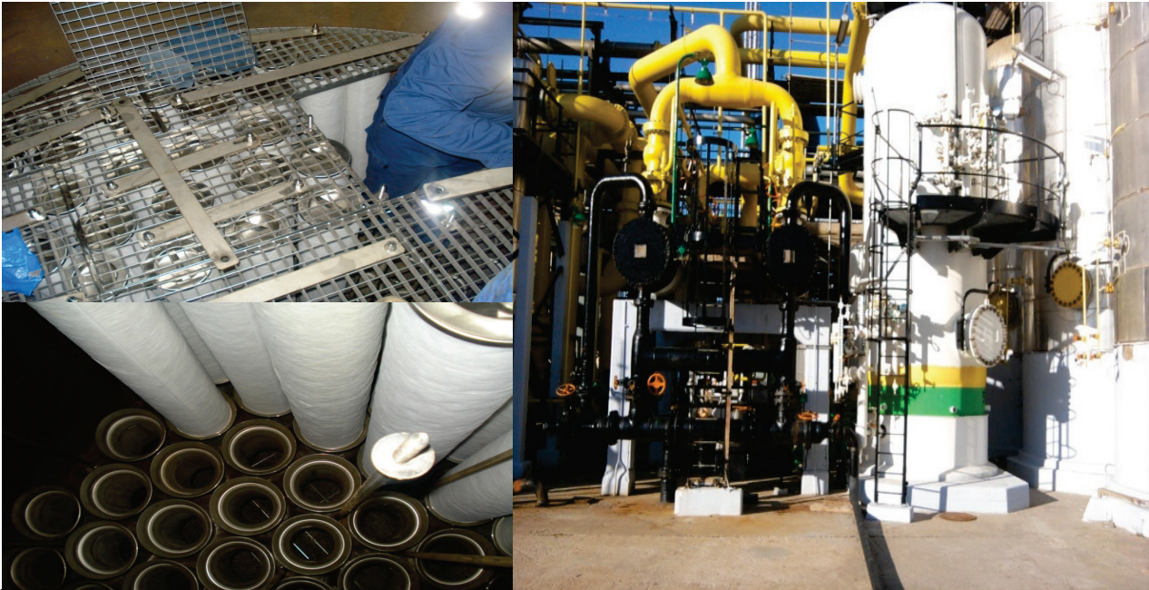
Figure 11: Installation of a new liquid-gas coalescer 61 D103A
