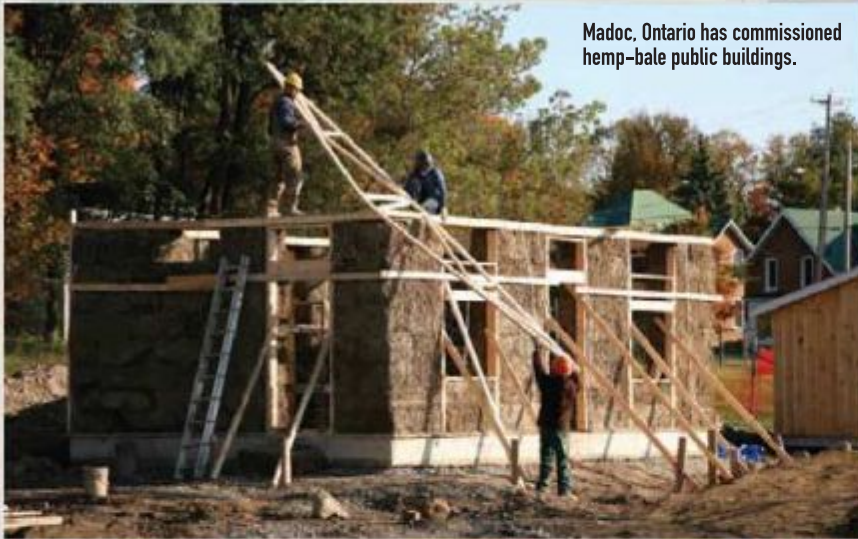
New hemp-bale structures are adjunct buildings to the new arts center (background).
