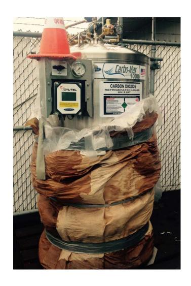
This tank is 1000 liters (according to this distributor these Doers are measured in liters. The CO2 conversion to get to pounds is 2.238 liters per pound or 8.79 cubic feet per pound
