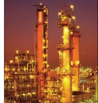
Process Heating and Cooling
